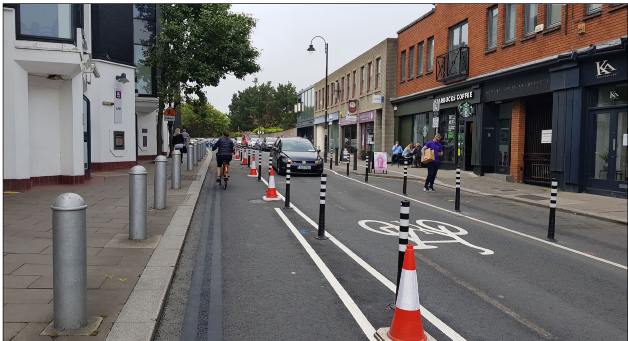
Figure 3.5: implementation of one-way system for vehicular traffic to provide additional space for pedestrians and cyclists.
