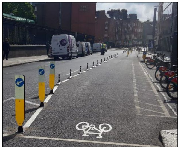
Figure 3.4: Segregated cycle lanes with plastic wands (Dublin City Council).
